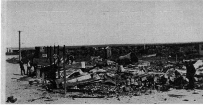
Aftermath of fire at Smith & Parrott's Store at 8.00pm on 13.8.1928.
